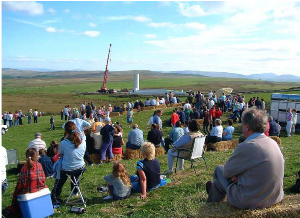
©T riodos. Locals gathering to watch the installation of the 1 st turbine at Moel Maelogan wind farm, Conwy, Wales
